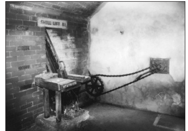
The shell lift remains in remarkably sound condition. Only the ingress of rainwater from above prevents the chains which operate it from functioning.
